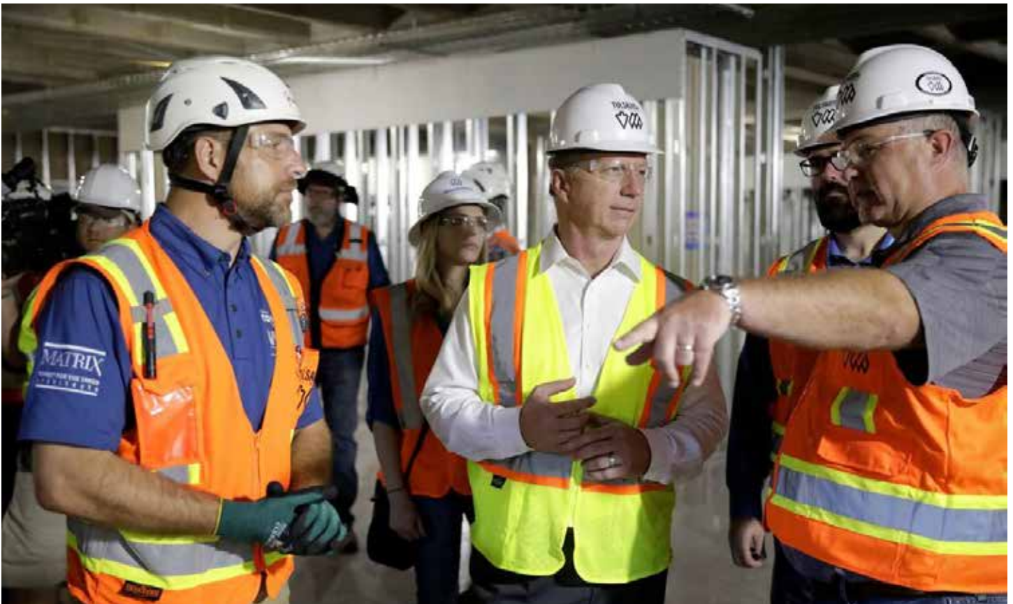
Oklahoma Congressman Kevin Hern gets a first-hand look at the construction of the Cox Business Center in downtown Tulsa. This project is a $55 million joint venture between Flintco and Manhattan Construction Company. Pictured from left to right are Flintco Sr. Project Manager Andrew Witte, Congressman Hern, Manhattan Sr. Project Manager Mike Flaherty and Manhattan Project Director Jason Martin.
