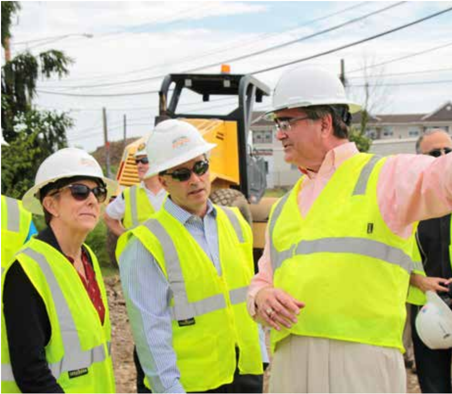
Ohio Congressman Troy Balderson (middle) tours Shelley & Sands, Inc.'s $32.7 million project in Columbus, OH that includes the widening of Lazelle Road and creation of a roundabout intersection along with the Chris Runyan, Executive Director for Ohio Contractors Association and Teri Geiger, Chief of Staff for Rep. Balderson.
