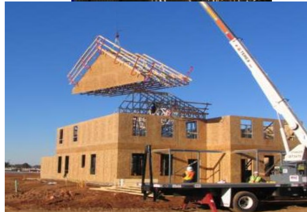
Properly assembled and braced IAW the manufacturer's instruction and the BCSI guide
