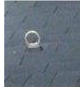
Wood Roof Anchor
