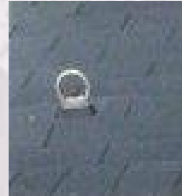
Wood Roof Anchor
