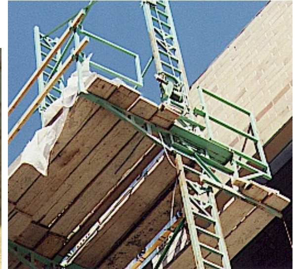
Ladder Tower with gate
