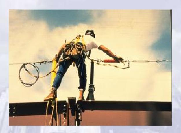
An example of proper tie-off at a connection
