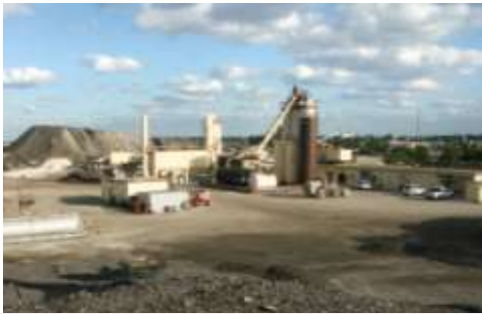
Ranger Construction Industries Photo: Asphalt plant showing piles of RAP, a recycled wash water system (left foreground, silver tank) and a recycled oil burner fuel tank (right central area).
