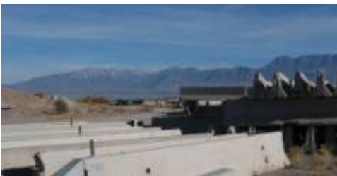
Ames Construction Photo: Stockpiled portable concrete barrier rails from a recently completed Department of Transportation Project in Utah County, Utah.
