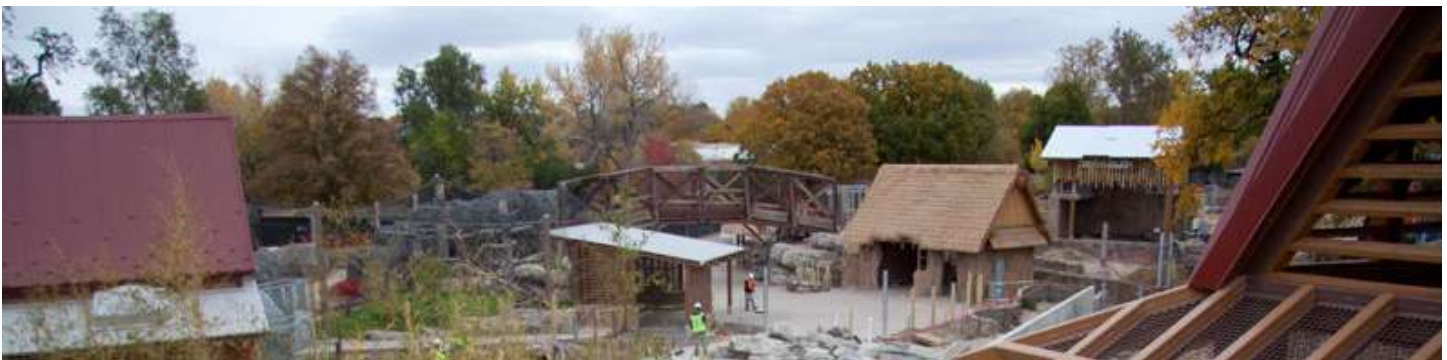
Kiewit Corporation Photo: Work at Denver Zoo Asian Tropics Exhibit.
