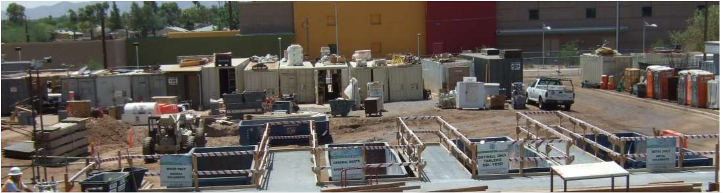
Kitchell Contractors Photo: Use of loading deck for recycling at Kitchell project.
